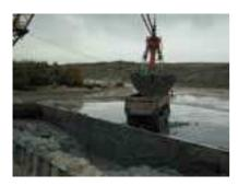
This project consisted of infrastructural works to dredge the West and South Industrial canals to a depth of 10.5 metres in order to improve the nautical accessibility in the port of Venice-Marghera. This will allow vessels of higher tonnage to access the port facilities and thus to develop maritime and comodal transport. Furthermore the project aimed at reducing the environmental pollution of the lagoon by removing the contaminated sediments from the two canals.
